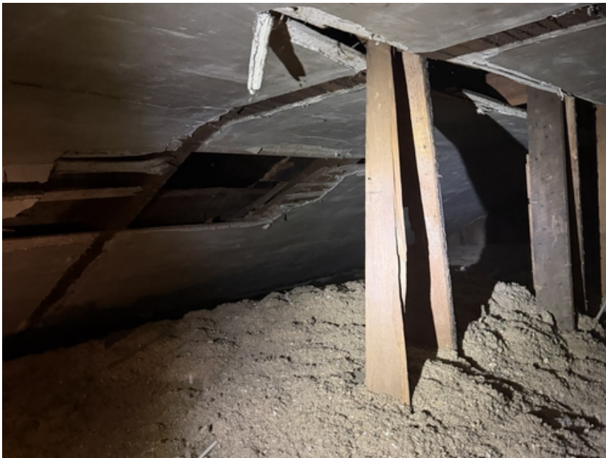
The attic section closest to the road shows an older ceiling system that will be ventilated on the upper pitch and through the other section of the library.
